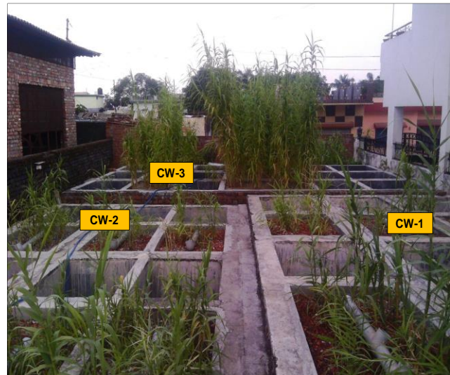
Fig. 1. Left: Schematic diagram of VSSF CW units; Right: Picture of CW-1, CW-2 and CW-3 near Graphic Era dairy farm.
